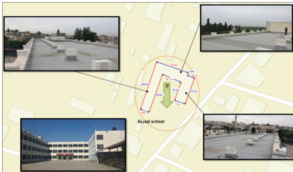
Figure 3: Al-Razi boys school top-roof building
