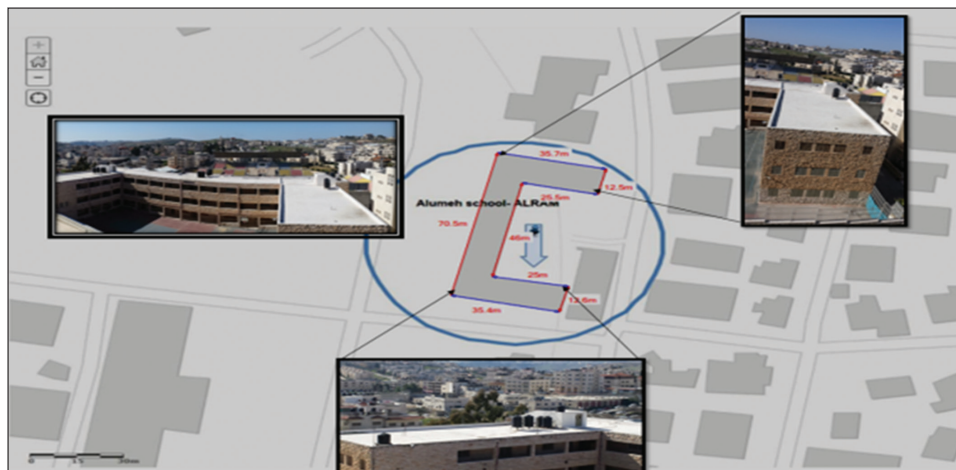
Figure 4: Al-Umeh boys school top-roof building
