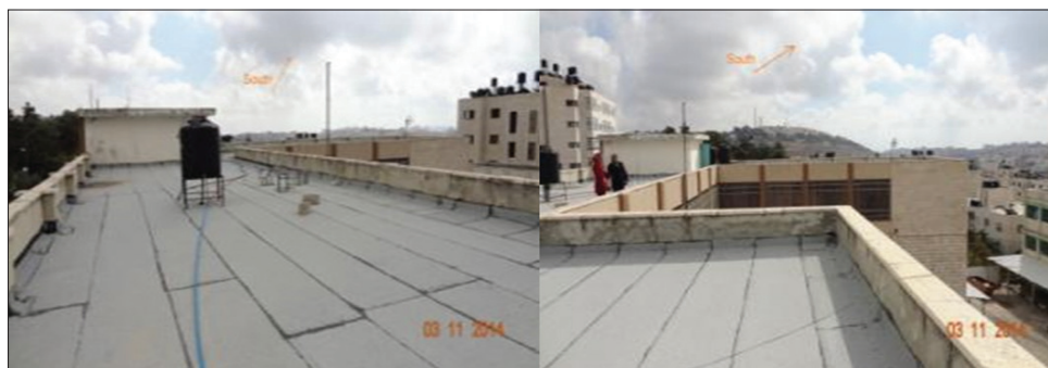
Figure 5: Khawlah Bent Alazwar girls school top-roof building
